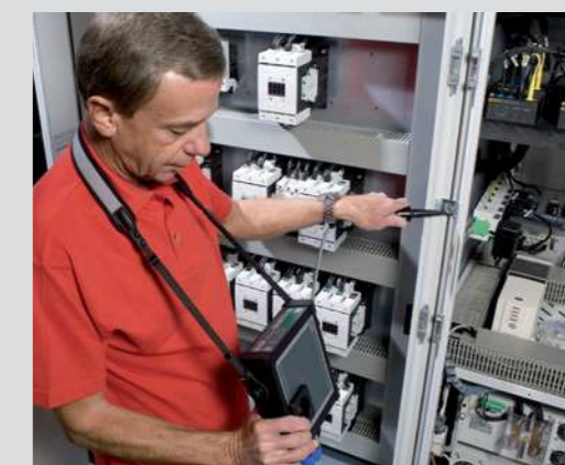
EN60204 test at a service cabinet
